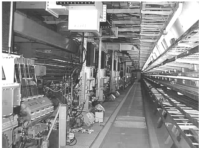
Fig. 4. HERA accelerator tunnel.
